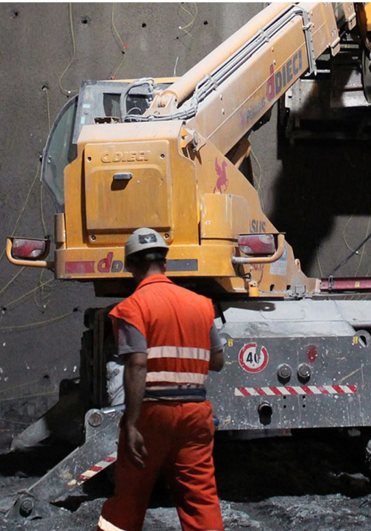
Workers opening a tunnel. Photograph taken by Malke and Björn Bröskamp.
